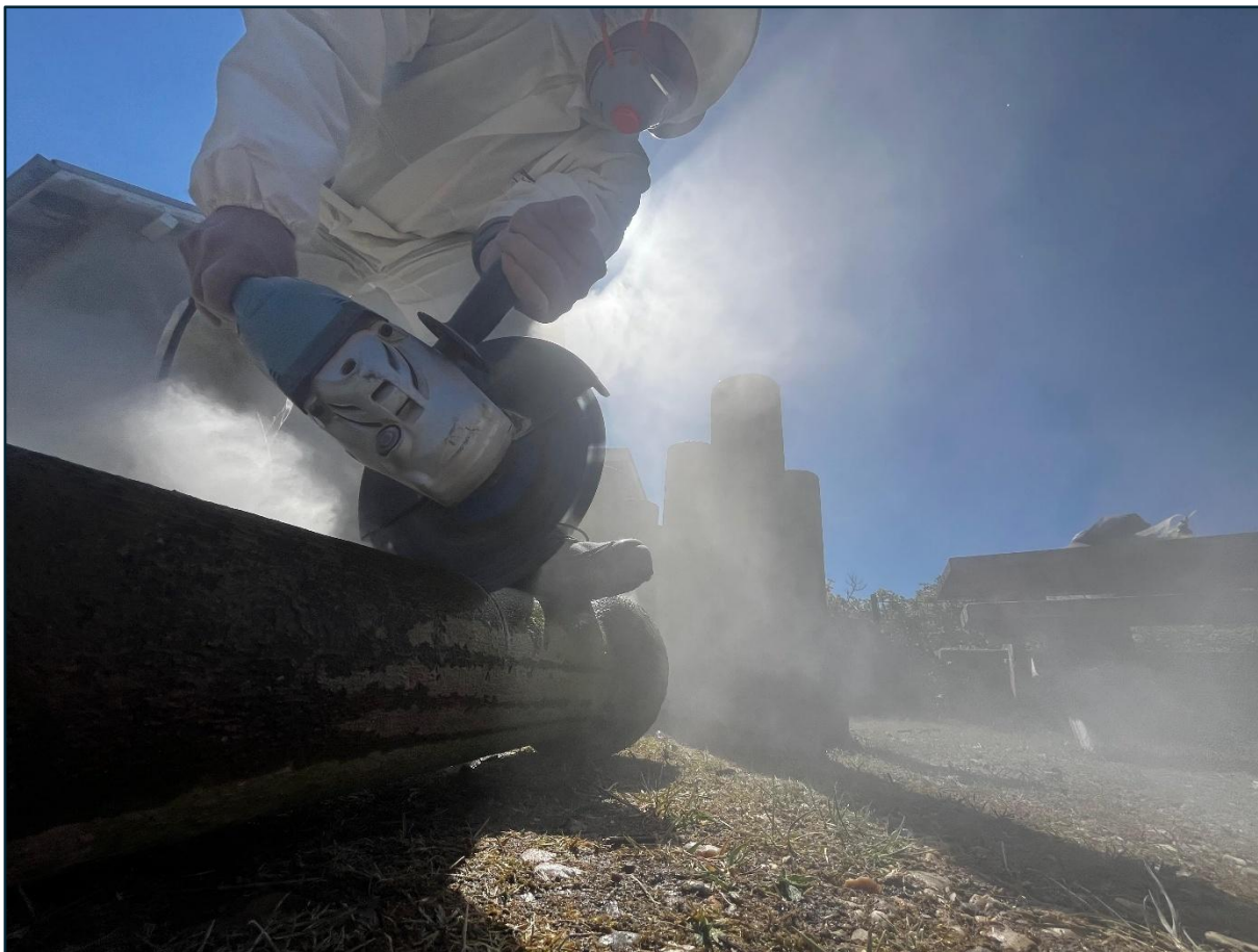
Appendix 3: Cutting concrete tubes
